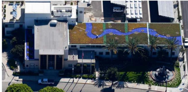
**Figure 2. Green roof on Burbank Water and Power Building.**
